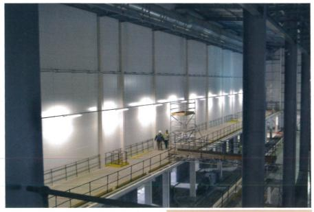
walls or whole buildings, offering fire resistance from 60 to 240 minutes where needed. ISD for example, has been successfully installing composite firewall systems to protect buildings and contents for over 15 years.
